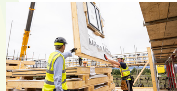
Sigma II Closed Panel Build System, Donaldson Timber Systems (formerly Stewart Milne Timber Systems)
