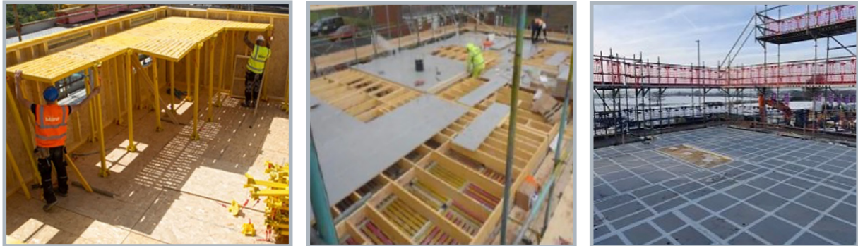
Figure 7. GEN1 Loose joists, safety decking and forklift installation
