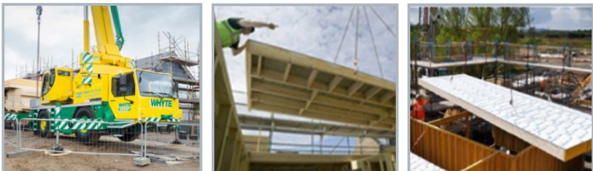
Figure 8. GEN3 floor cassettes, no safety decking and crane installation
