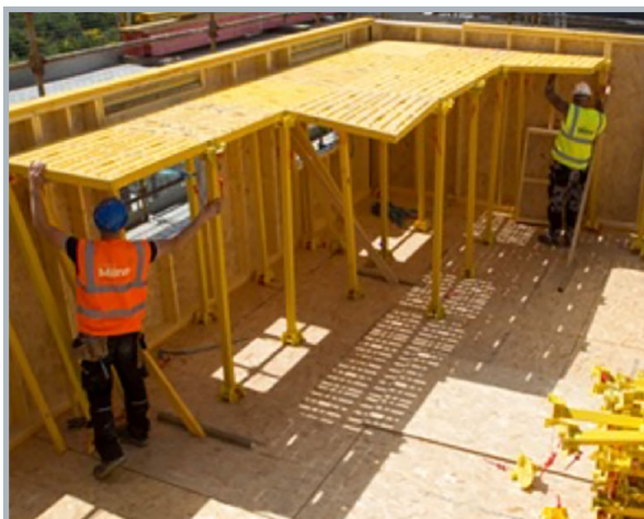
Figure 10. GEN1 Loose Joists Construction Method
