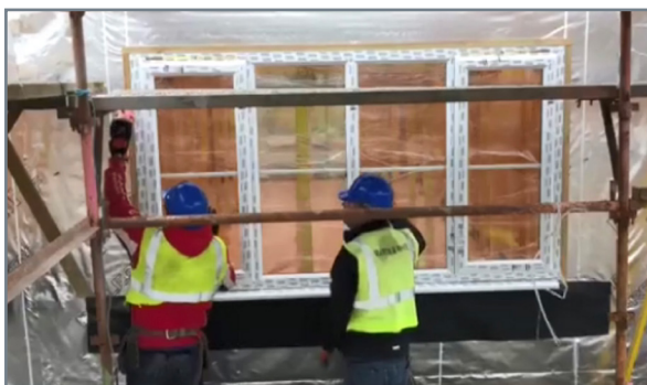
Figure 19. Site v Factory Nailing Process, Reach and Access
